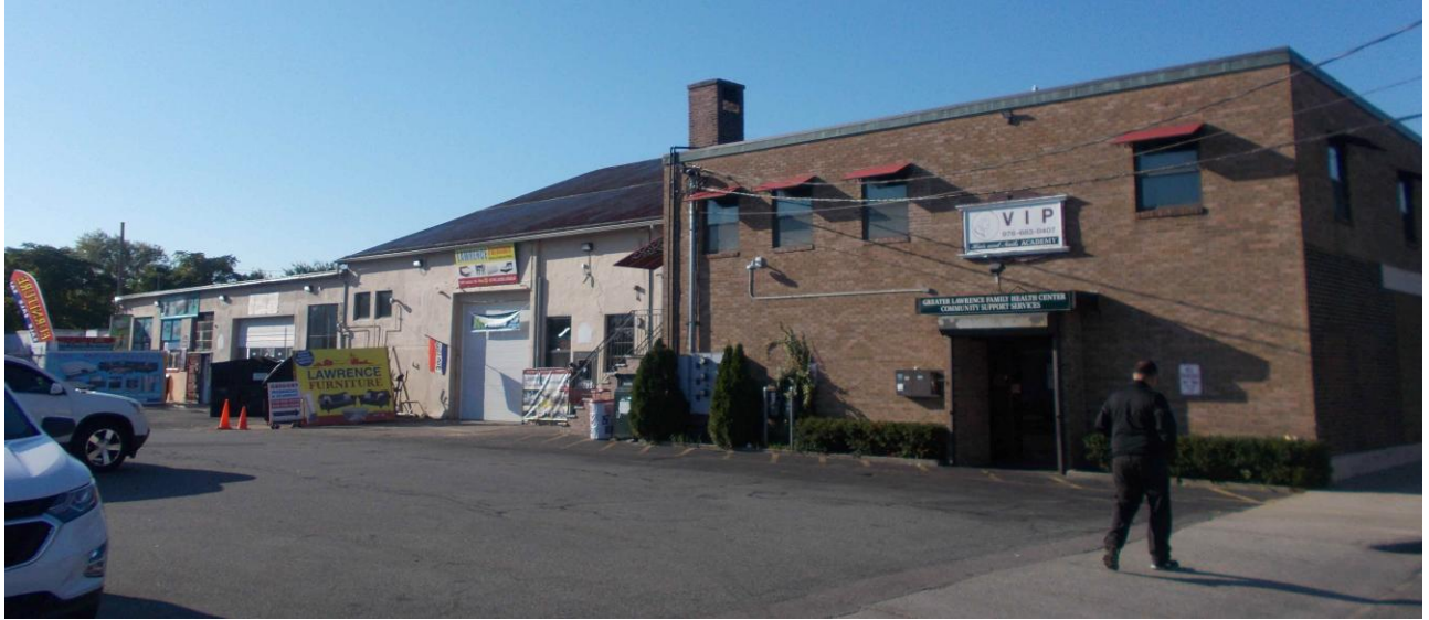
Figure 3: Photo – Existing Multi-tenant Buildings at 100 Water Street, Lawrence, MA (source: tax record photo, September 26, 2019)
